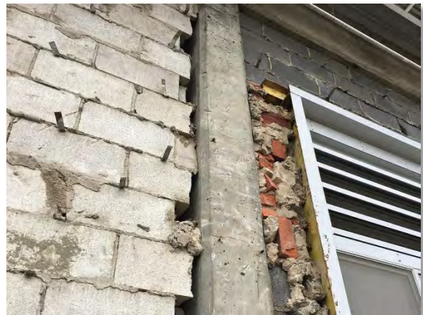
Figure 2 - Headworks Siding Removed
