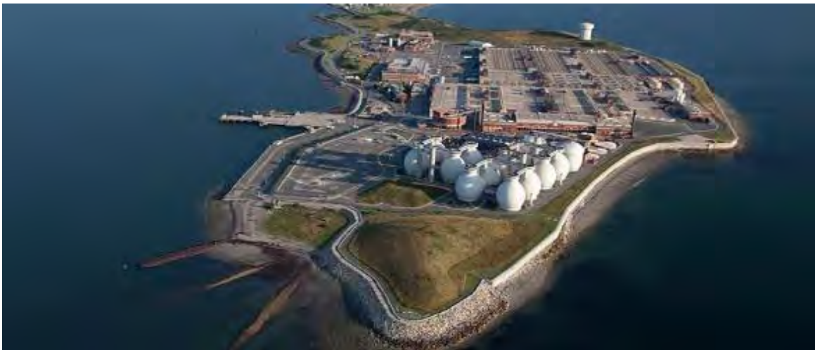
Deer Island Wastewater Treatment Plant
