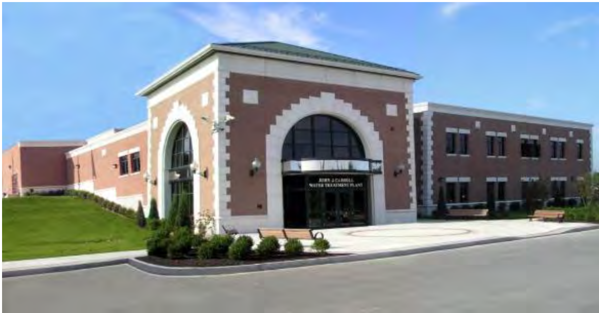
John J. Carroll Water Treatment Plant
