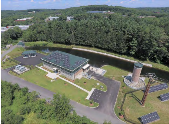
Figure 3 – Wachusett Aqueduct Pumping Station Zero Net Energy
